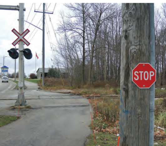
Top left: Active warning system with gates. Centre: Passive warning system on a low-speed roadway in an industrial area. Right: Example of an active warning system without gates that would benefit from better delineation, sightlines, and the installation of stop bars for active road users.
